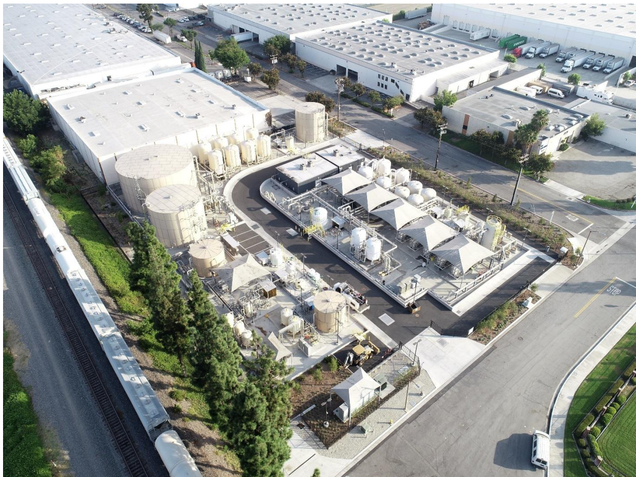
Figure 2 – PVOU-IZ and SZ Treatment Facilities
