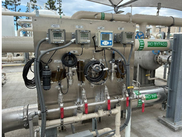
Pre-RO Analyzer Panel (AIT-2145 & AIT-2155 probes replaced)
