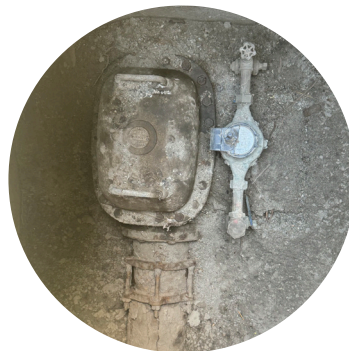
Single Check Backflow Prevention Assembly
