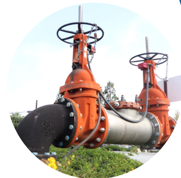
Double Check Backflow Prevention Assembly
