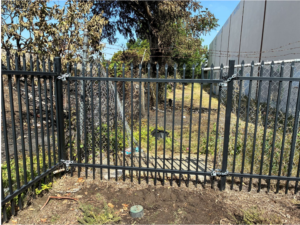
Short-Term: Temporarily Affix Fence Panel
