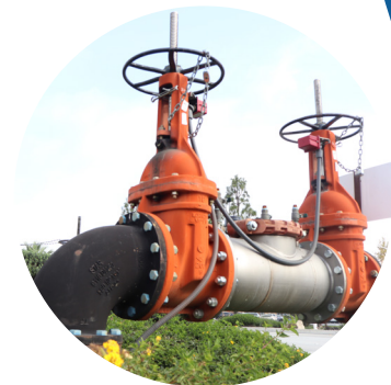
Double Check Backflow Prevention Assembly
